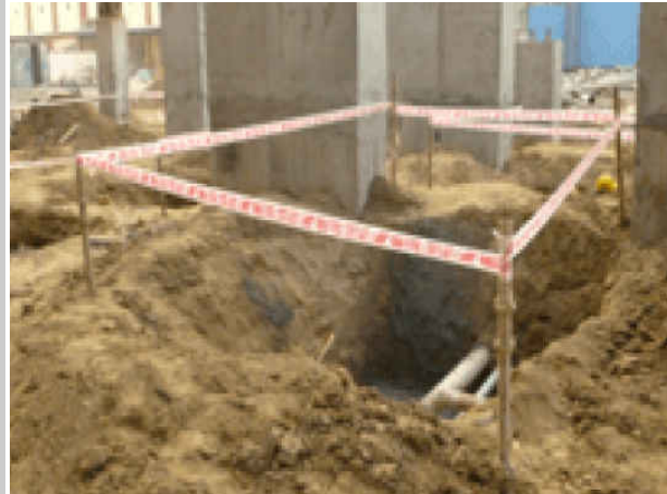
FOUNDATION BARRICADING
